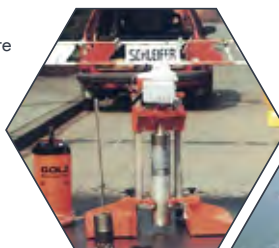
Drilling out water valves (Ø 200 mm / 8")
